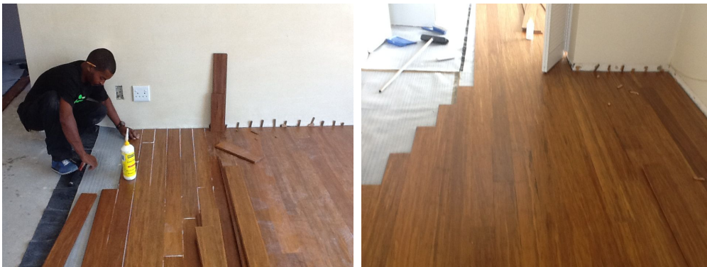
Tongue & groove planks installation above
