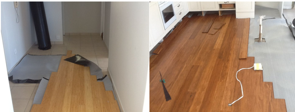
Click planks installation above (glueless)
